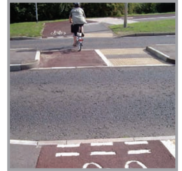
Central island crossing, National Route 1, Sittingbourne to Canterbury
