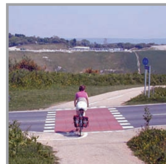
An uncontrolled greenway crossing of a road, National Route 3, Eden Valley
