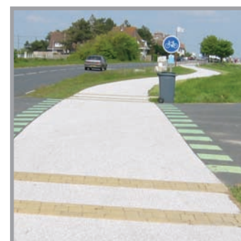
Rumble strips on the greenway approach to a road
