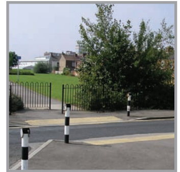
Cycle route crossing of a minor road, with buildout and priority working for vehicles, National Route 65, Hull
