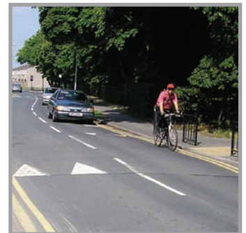
Raised crossing point where a greenway crosses a road, National Route 65, Hull to Hornsea
