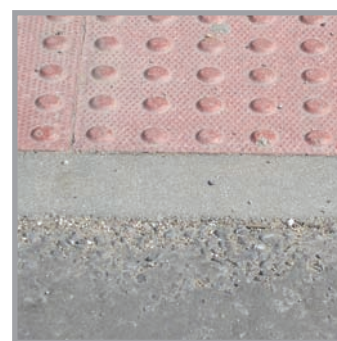
Flush kerb detail at a Toucan crossing
