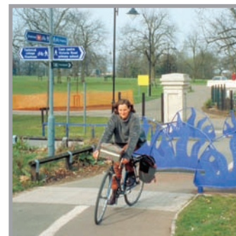
Effective chicane incorporating artwork to reduce cyclist speeds approaching a road crossing, National Route 15, Nottingham to Skegness
